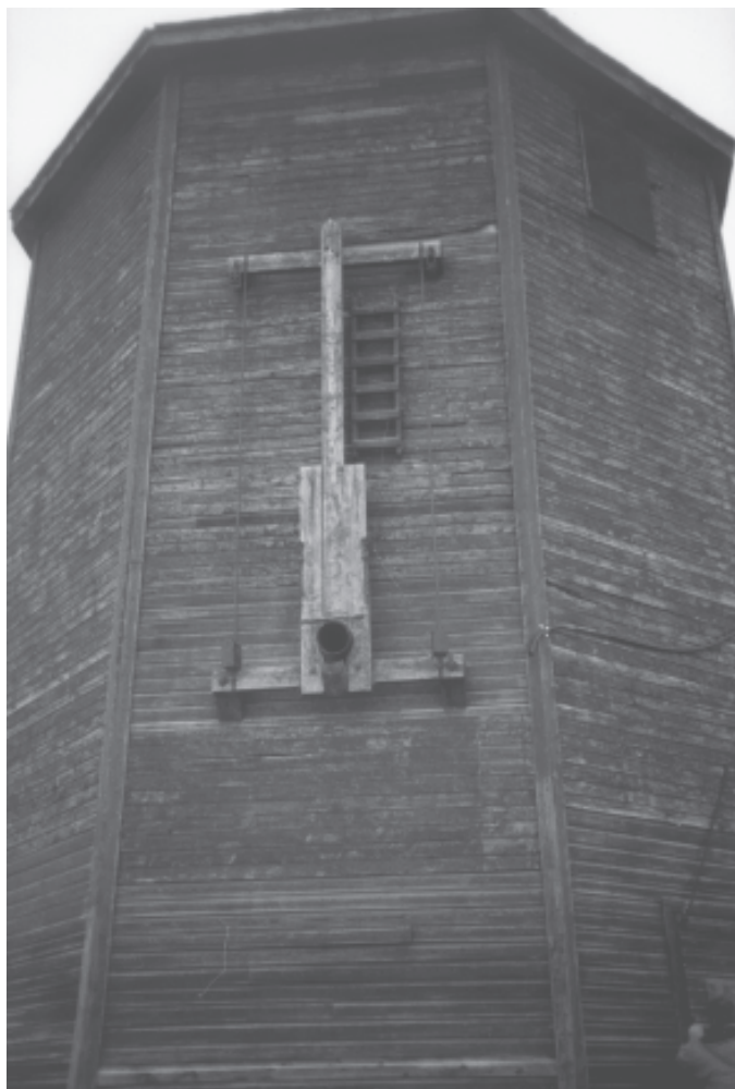
The water spout on the tower which filled the locomotive with its' supply of water.
