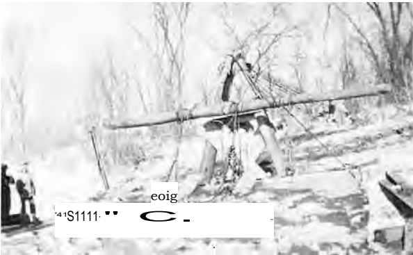
In 1948, the maintainer sank through the ice. A tripod winch was used to pull it out.
