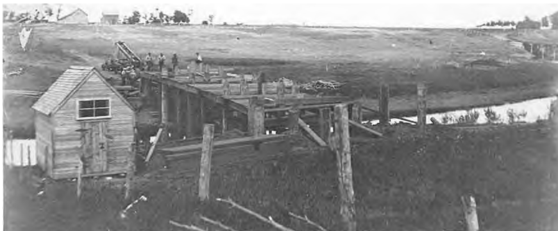
Municipal bridges were a great necessity, to cross the Morris River that winds through the municipality, and to traverse the drainage ditches. This bridge at Rosenhoff was built by Jacob Penner (bridge foreman) under contract for $550.00 in 1936. Pile driving was done manually, and the dirt work done by spade - no backhoes then.
