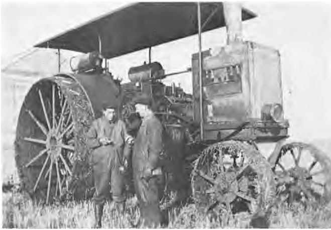
Ray Loving and engineer W. Kelly with Auliman - Taylor tractor, 1916. NOTE: Gas head lamps and drive wheels 3 ft wide and 8 ft high.
