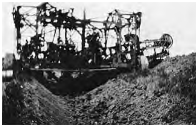
Ditching machine at work on the Bell Drain. Photo courtesy Walter Anderson.
