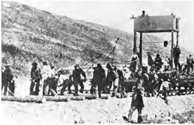
Early construction of the CPR on the prairies in 1882. Here showing the section gang laying track. Photo courtesy Manitoba Archives.
