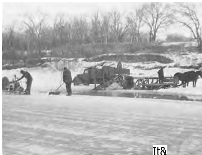
Snarr's ice outfit on the Red River in the 1950's. One man is clearing snow, while the other is preparing to use the saw. Horse and wagon await another load. Ice harvesting was discontinued soon after this time.
