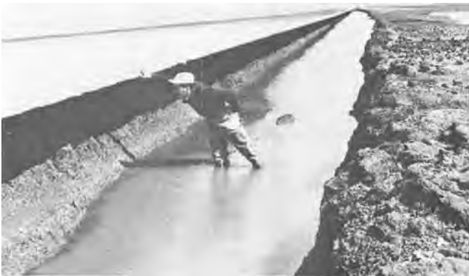
Highways Dept. inspects the damages created by the erosive effects of wind and waves on this paved highway. Courtesy Manitoba Archives.
