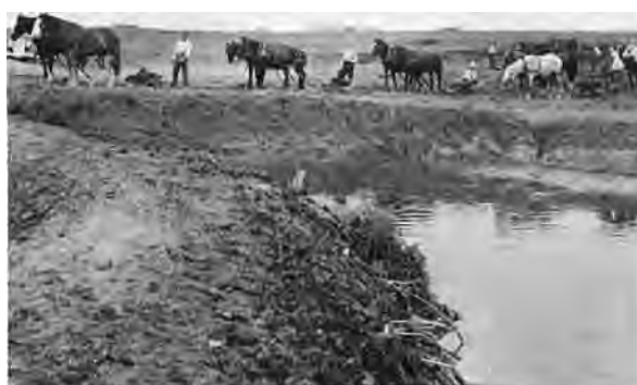
Damming the Morris River at the George Bartel farm, to build a pond for livestock.
