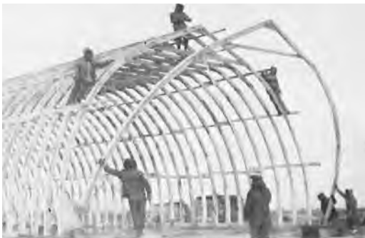
The last rafter going up on a 32' X 160' rink. Over 2500 pieces were used to make the rafters.
