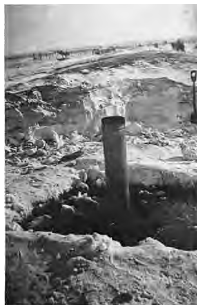
One way to keep a supply of water on hand throughout the winter was to immerse a stove in a water tank. (E.F. Lewis farm).
