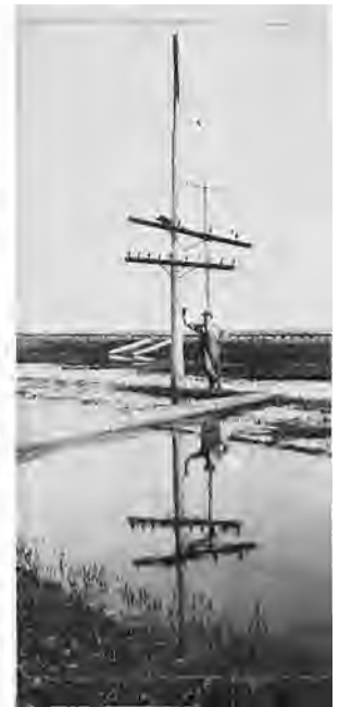
RIGHT: James Smith, telephone districtman, repairing poles in 1927, which were broken in a sleet storm. Photo taken near railroad enroute. Lowe Farm.
