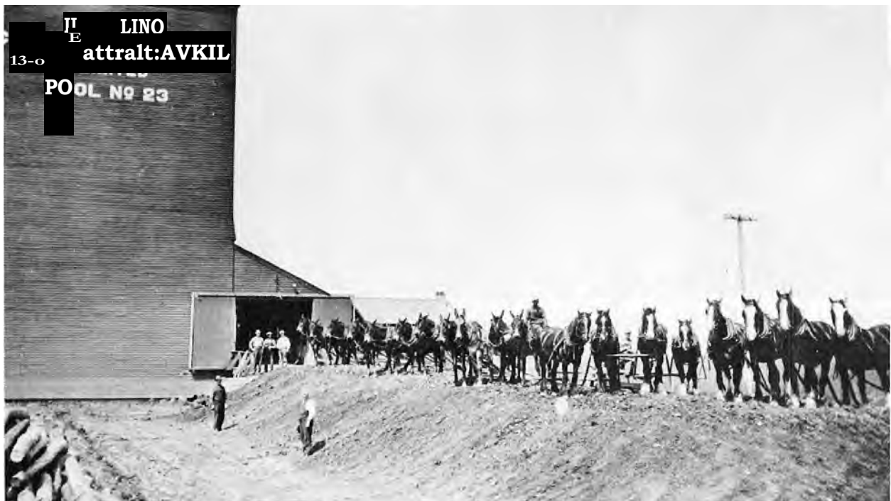
Mules and horses combined, provided the draft power for the road scrapers in constructing the driveway to the first Pool elevator at Sperling in 1926.
