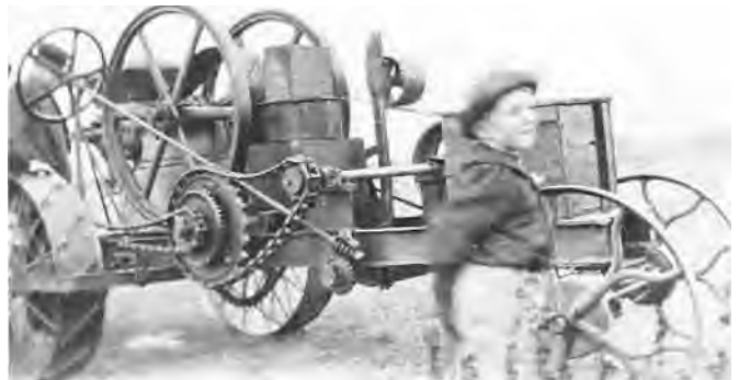
D.K. Kroeker's homemade tractor, constructed in 1915 by a blacksmith, Mr. Buyan. Rear wheels of binders, front wheels from grass mowers, clutch either by belt or spider drive. David Kroeker behind tractor and P.L. Kroeker in front.
