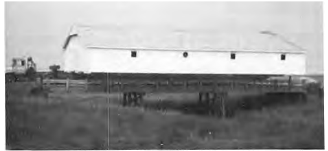
Dueck the movers, moving a barn. The barn had to be raised in order to clear the posts on the bridge.
