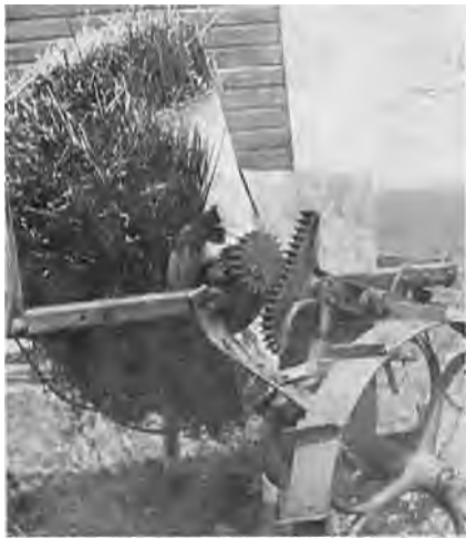
Stooking machine, invented and patented by John I. Dyck about 1927.
