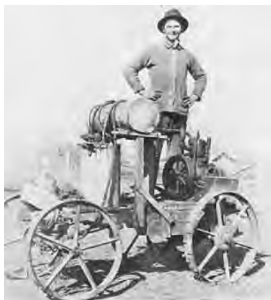
Wm. Poersch in 1912, with a small tractor he built from an old grass mower chassis. It was used for small jobs on the farm.
