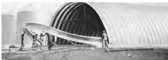
Here, the steel machine shed under construction. It was completed in 3 days.
