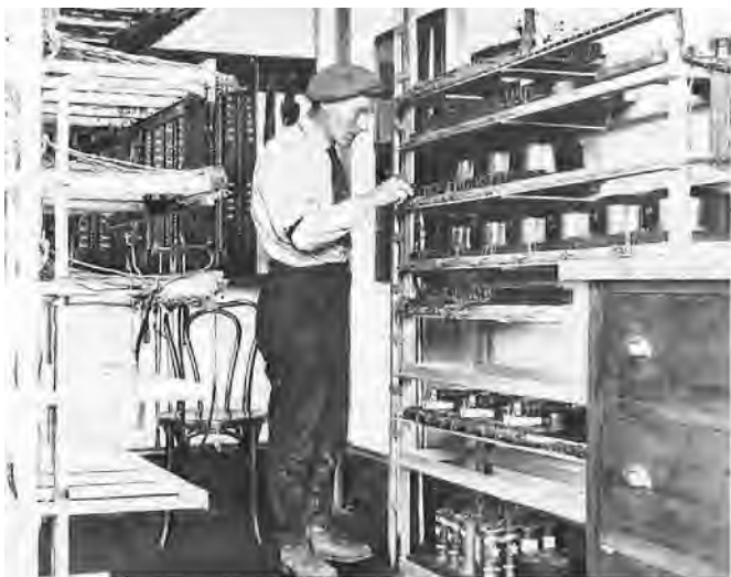
James Smith in telephone office rack room working on phantom coils, a method used to have three conversations on four wires. Taken in the 30's.
