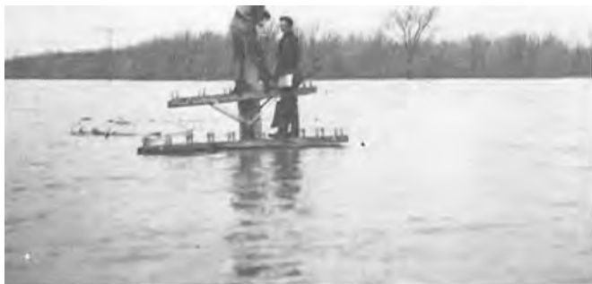
Telephone linemen adding extensions on to the poles to raise the lines (1950).
