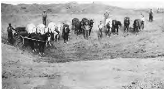
Until the advent of the dragline, dugouts were excavated with horses and slush scrapers. This picture shows Peter U. Braun and Peter P. Harder using their horses and plow to loosen soil, while sons, Peter and Jacob Braun, and Peter G. Harder, Jacob Froese, and Cornelius Driedger Jr. removed the soil with horses and scraper. Dugout was being made at Peter P. Harder's farm in 1931.
