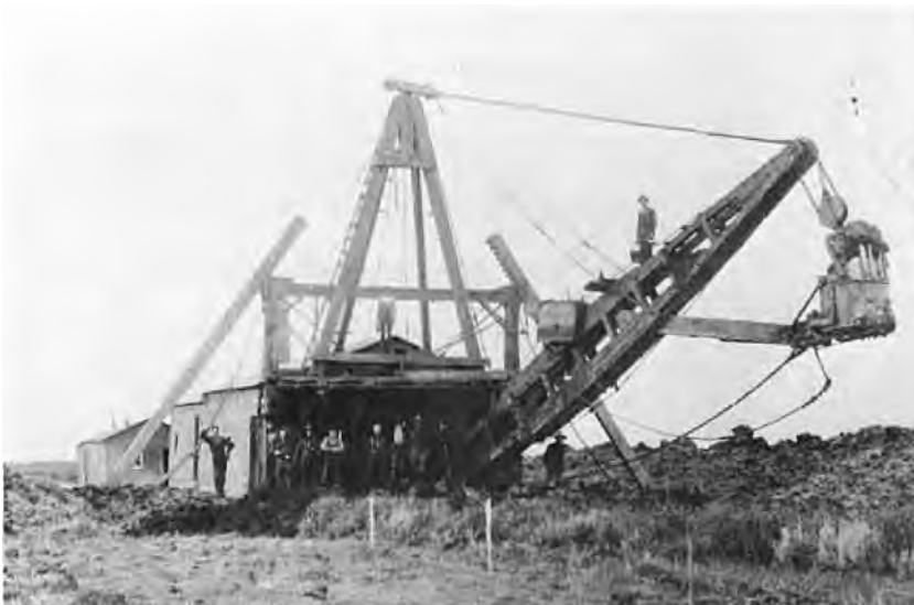
LEFT: The floating steam dredge that dug the Tobacco Creek drain in 1903.
