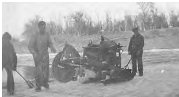
Gottfried Boggs and Ewald Dreger cutting ice with a saw built from an old car motor. (1943)
