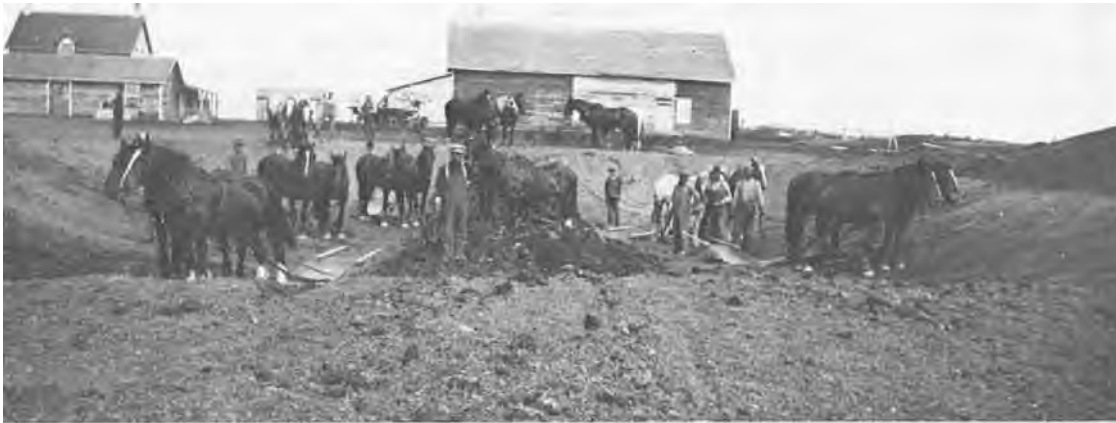
Farmers with their teams using slush scrapers, often were required to do the road building. This gang is digging a pond at the C.A. Recksiedler farm.
