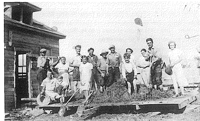
Mixing clay Plaster (a mixture of clay and straw) for walls of Steve and Elsie Trakalo's home (1938). Front Row: L to R: Teenie Trakalo, Elmer Trakalo, Ann Shmyr, Ernest Trakalo. Back Row: L to R: John Shmyr, Mary Glushka, Pete Leschasin, Willie Antonichuk, Sam Trakalo, Pete Skoncylas, Nellie Shmyr, Ann Womitoway, Steve Trakalo, Thelma Leschasin.
