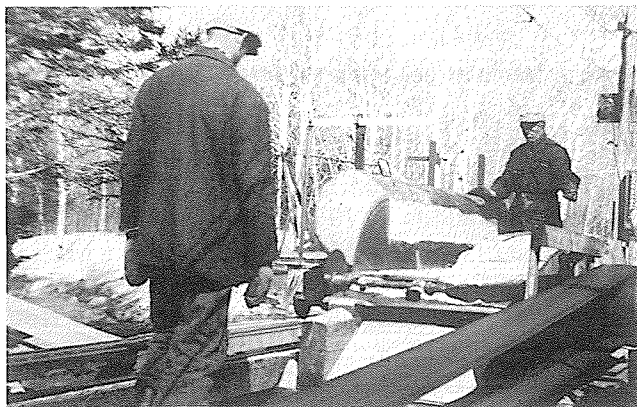
Joe Kryswaty and Mike Topolnisky sawing logs. Note the central panel and string of wires mounted on pole behind Mike. This enabled Mike to control operation of tractor and sawmill from his sawyer's position. Photo taken in late 1950s.
