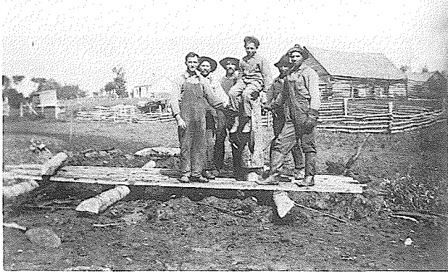
Sitting on a "tile drive" block of wood with 4 handles used by 4 men to drive the posts into the ground. Left to right: Fred Topolnisky — holding jug, Willie Antonichuk — holding spade, John Antonichuk — holding saw, Allan Elvers — holding saw, Otto Elvers — axe, John Levitsky — with straw hat, Bill Kalyniuk — black hat, Wasyl Antonichuk — by tile drive.
