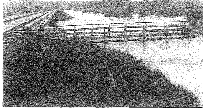
Brightwell's bridge washed up against CN Railway bridge at Birdtail at the peak of a flood of the Birdtail Creek (1940's).
