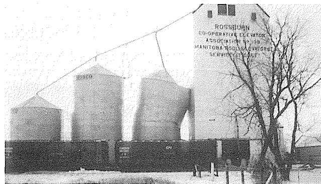
A steel annex at Rossburn Pool Elevator burst on Nov. 28, 1967 spilling a quantity of grain on the ground and on the tracks. The annex buckled about two-thirds of the way up. Fifteen thousand bushels were in the annex at the time of the incident.
