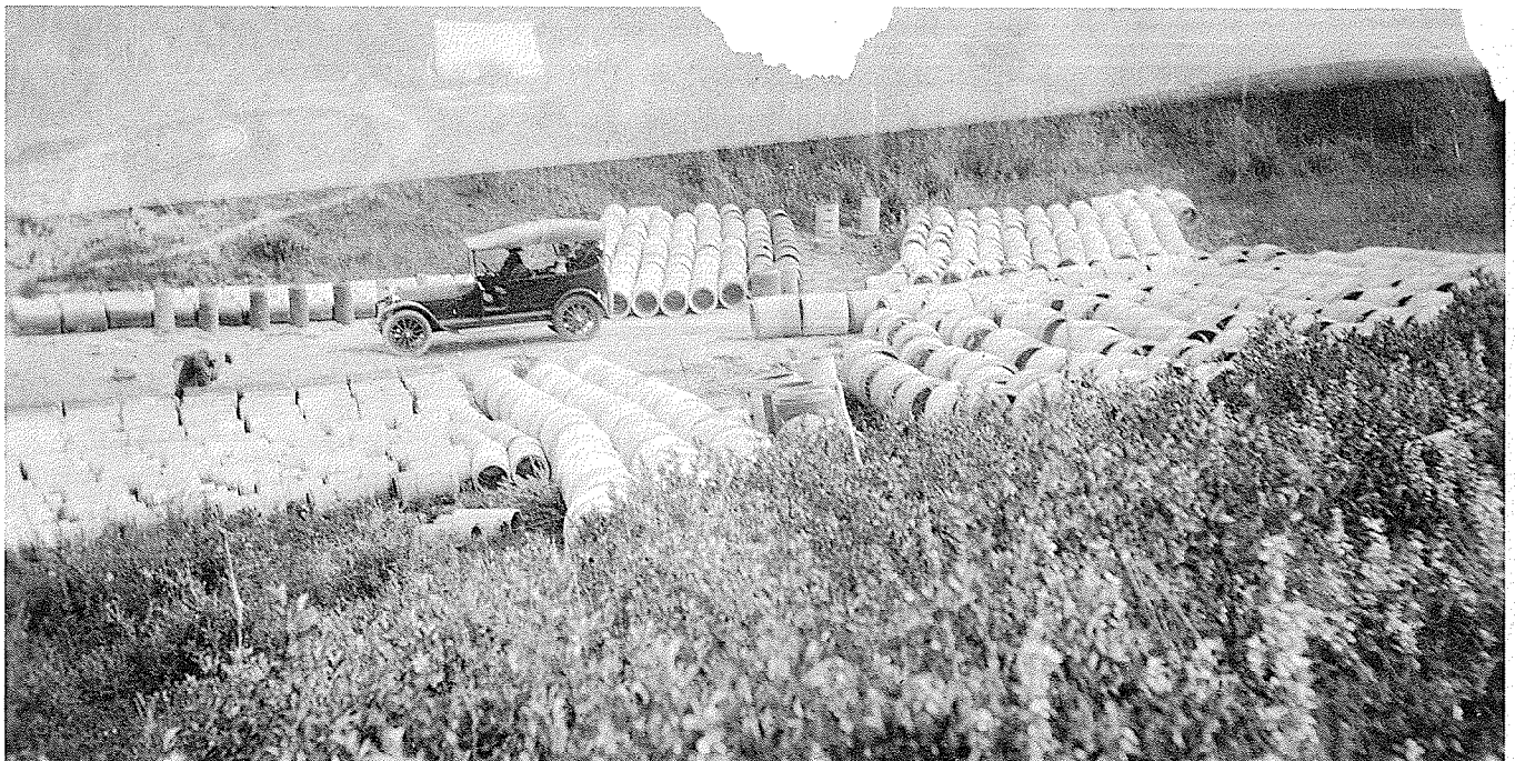
Construction of Cement Culverts to be used in the building of roads in Ellice Municipality.
