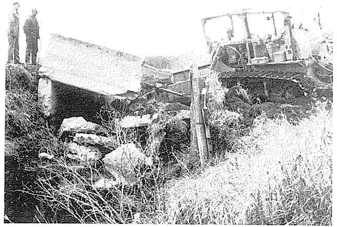
Old bridges were built solid but eventually had to give way to new concepts so the old cement bridge between sec 2 & 3 -9-17 had to come out to make way for a large metal culvert.
