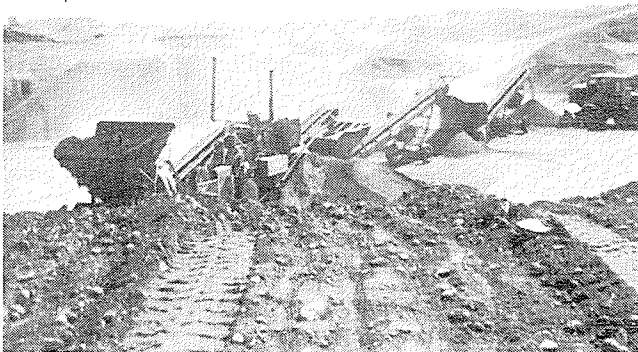
Modern machinery and methods greatly aid the development of better roads. Here activity in the Harris gravel pit processes traffic gravel and below crushed stone for firmer road bases.
