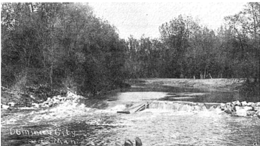
The C.P.R. dam (behind the present home of W. A. Taylor) ensured the railway of a good water supply for the old steam engines. Also, it was hoped that the lower water level to the left of the picture would steady the bridge piles and prevent them from shifting.
