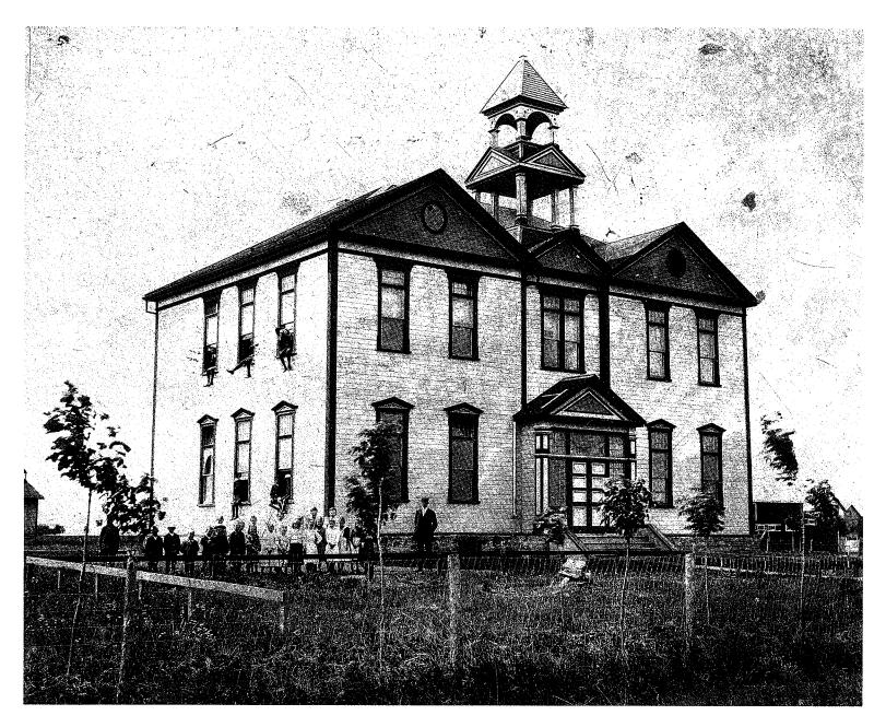
This two-storey frame schoolhouse was built in 1899 for \$7,000, and dismantled in 1938. A bell in the bell-tower summoned students from Grades 1 to 12 to the four-room school (two classrooms on each level). It was located on 3rd Ave. NE where the Elmwood Apartments were built in the 1980s.
