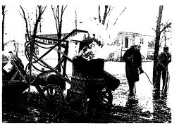
Drainage during the spring thaw was a perennial problem during the 1950s, when heavy snowfall marked the Manitoba winters. Here the public works crew employs a crude but effective steaming device that applied steam to frozen culverts to speed thawing.
