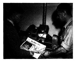
Installation of a Scan-a-graver in November, 1954, was a major event in photo journalism for the Echo. It enabled the paper to produce plastic halftones in a matter of minutes. Combined with modern darkroom equipment, the large number of pictures that started to appear in the Echo greatly boosted the paper's circulation and effect. Shown here with the new machine are Vic Penner, Echo editor (left), and Pete Wolfe, shop foreman.
