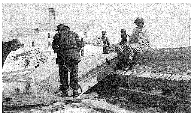
Reconstruction of wharf in March 1952 — placing the ice-shear along north side.
