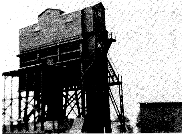
New coal dock built in 1928.
