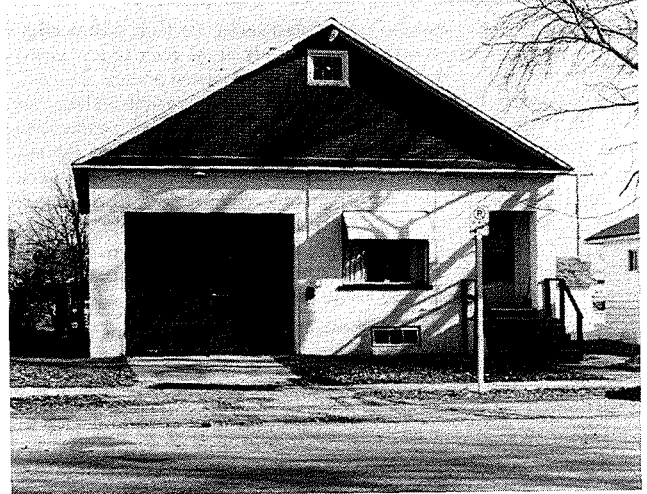
Village of Elkhorn Municipal Office, elevation — 1638 ft.
