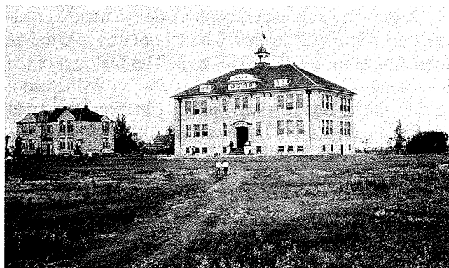
Elkhorn old stone school and new brick school 1910.
