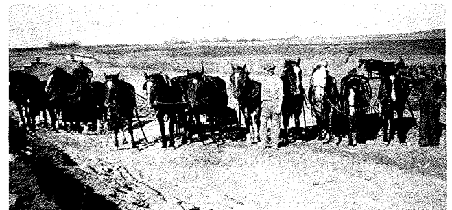
Bill Stonehouse's road gang, when building old No. 1 Highway, near Kirkella, 1931. Cliff and Morgan Shepherd by horses. Dannie and Alex Stonehouse also present.
