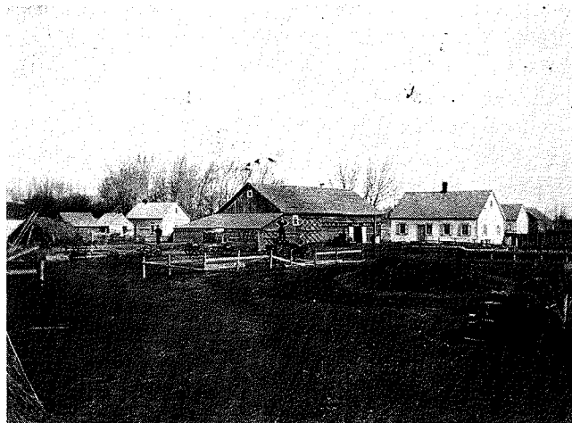
Many of the homesteads along the south side of the village street were built with the house and barn at right angles to each other whereas on the north side of the village the house-barn combinations were constructed in one continuous line. This yard at one time belonged to the Peter Peters family. It is presently owned by Abram H. Klassen.
