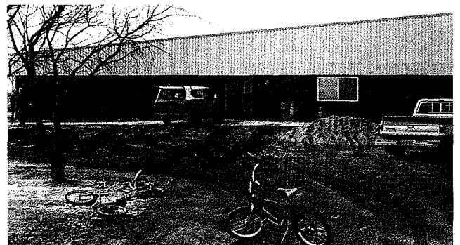
Side view of construction of the new building, 1982.
