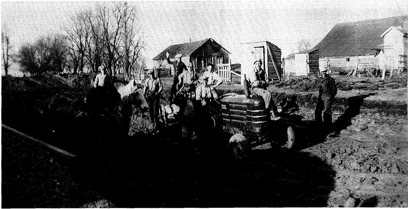
Digging the basement for the Gnadenthal church, 1942.
