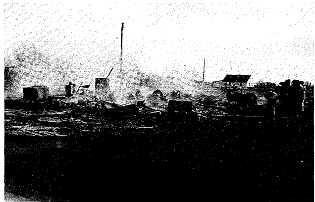
The Friesen garage was destroyed by fire in 1954.
