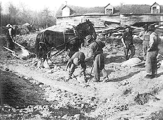
Basement excavation — with teams and slush scrapers.
