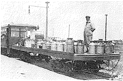
The "Mack Car" the front is closed off for the engine room, the back is for passengers.
