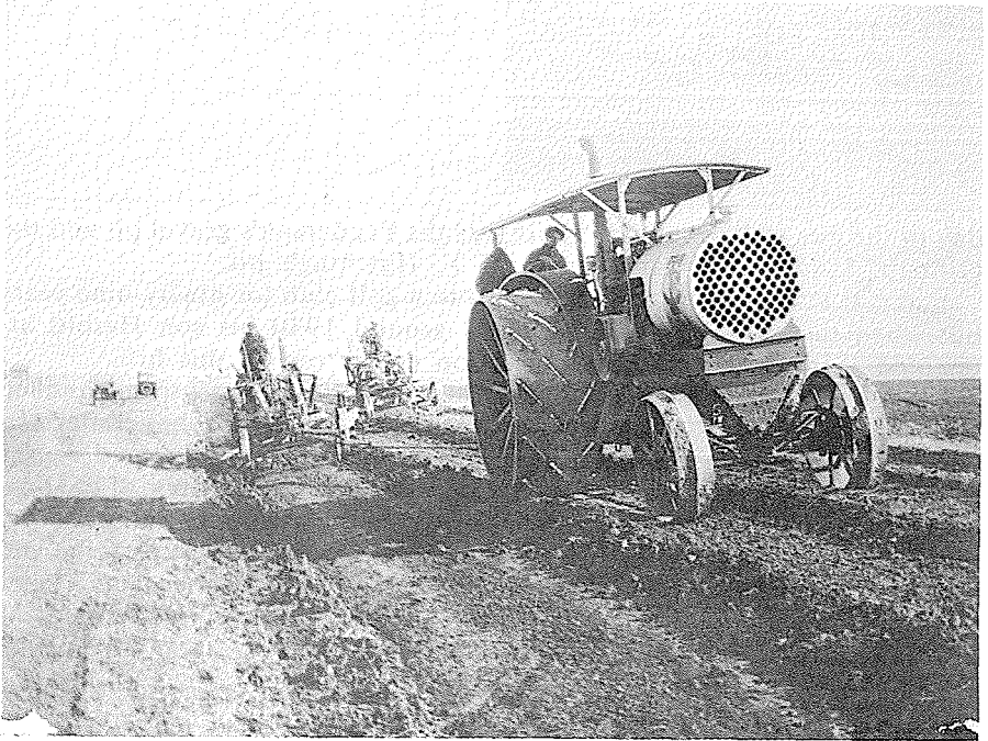
Twin City tractor 1923 constructing Dugald Road.
